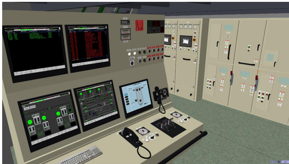
Unitest DE3D simulator. Engine Control Room with main switchboard of Platform Supply Vessel
