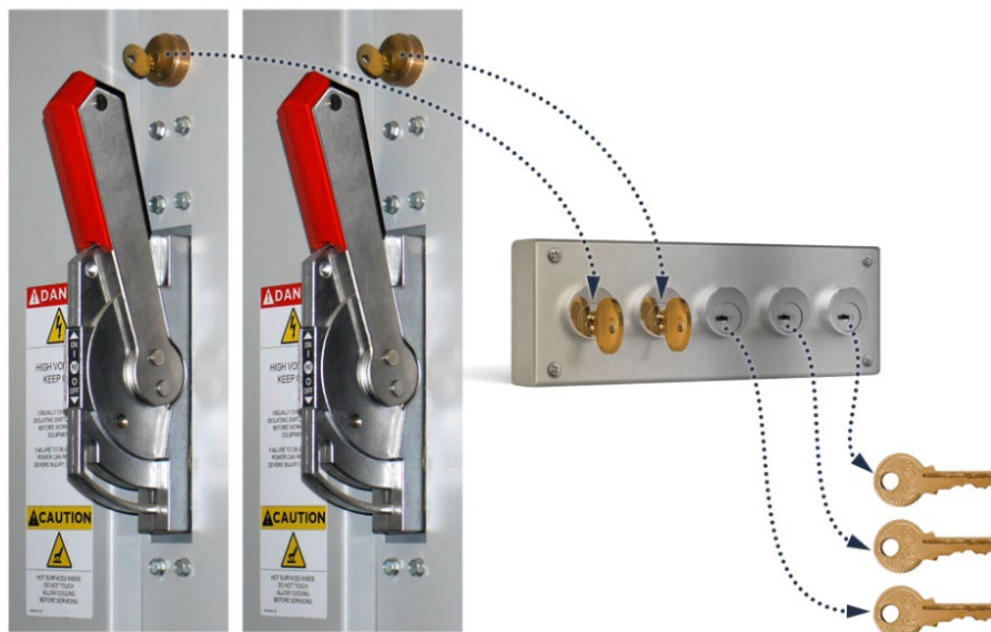
Three steps of trapped key interlocking.
